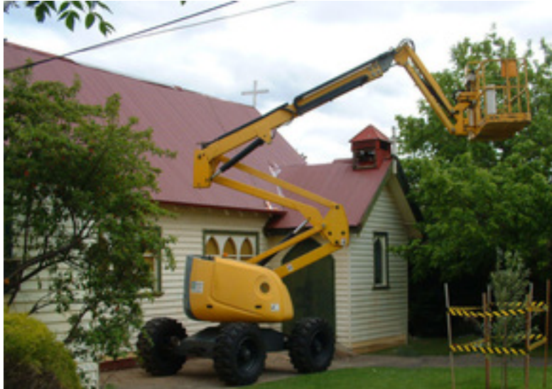
Cherry picker to put on capping November 2013.
